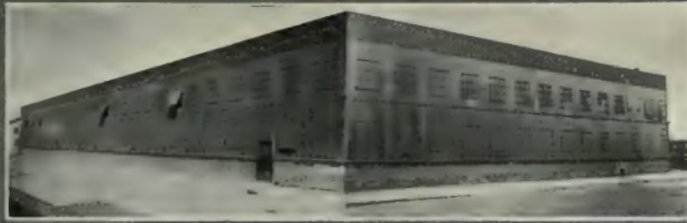
Exterior View of Assembling Department
