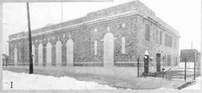
A. ROSELAND SWITCHING STATION 220-Kw. CIRCUIT BREAKER B. SUPERVISORY CONTROL PANEL AT W. 238TH ST. STATION, NEW YORK EDISON CO. C. SPERRY GYRO PILOT "METAL MIKE" D. HUDSON AVE. STATION, BROOKLYN EDISON CO. —Photo by Air Map Corporation of America
