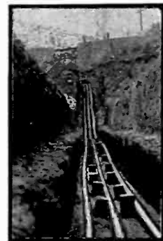
Cables in ground prior to back filling.
