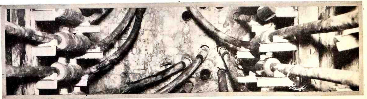
An installation of the Murray Cable Splicing Sleeve described above. Please mention the JOURNAL of the A. I. E. E. when writing to advertisers.
