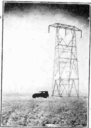
FIG. 10—COMPLETED SECTION OF LINE ON STANDARD TOWERS WITH EXTENSIONS
