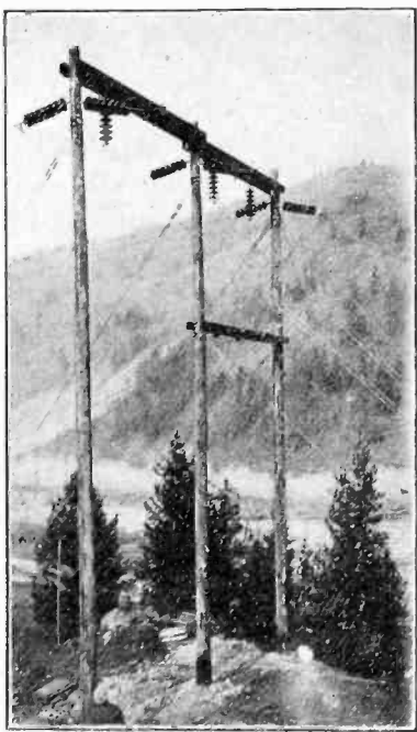
FIG. 13—TYPE "O", THREE-POLE STRUCTURE
