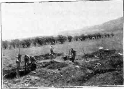
FIG. 7—SETTING TOWER FOOTINGS
