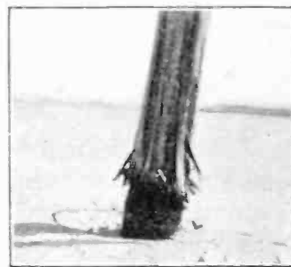
FIG. 5—POLE CUT BY ACTION OF ICE
