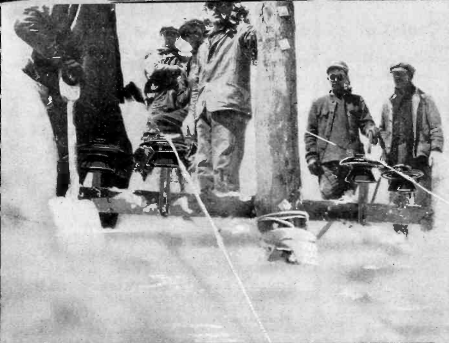
Locke insulators on the lines supplying power to the Moffat Tunnel near Denver.
