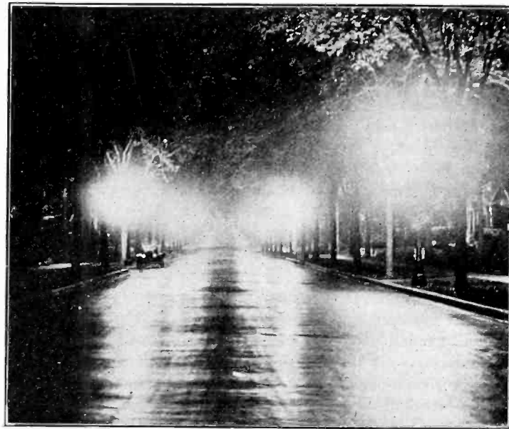
FIG. 1—HARRISON BLVD. SOUTH OF ARMOUR BEFORE AND AFTER NEW SYSTEM WAS INSTALLED. Spacing—Lineal feet of street per post—200 ft.—600-c. p. lamps—old system, 100-c. p. lamps.
