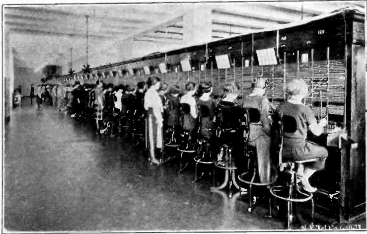
FIG. 2—MODERN TYPE COMMON BATTERY SWITCHBOARD
