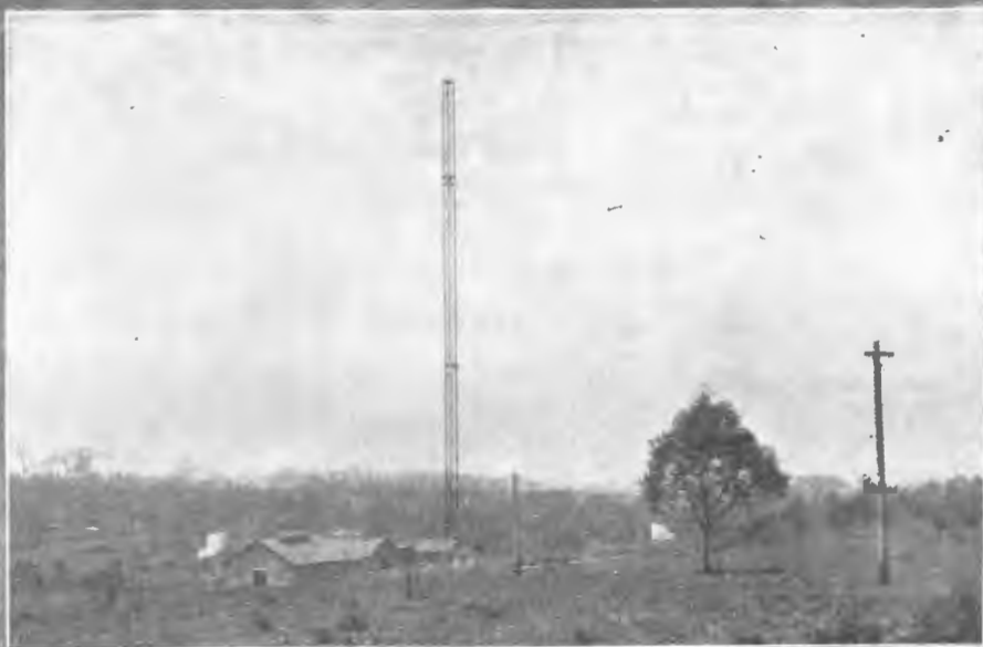
400ft. Mast at Pennant Hills, Sydney
