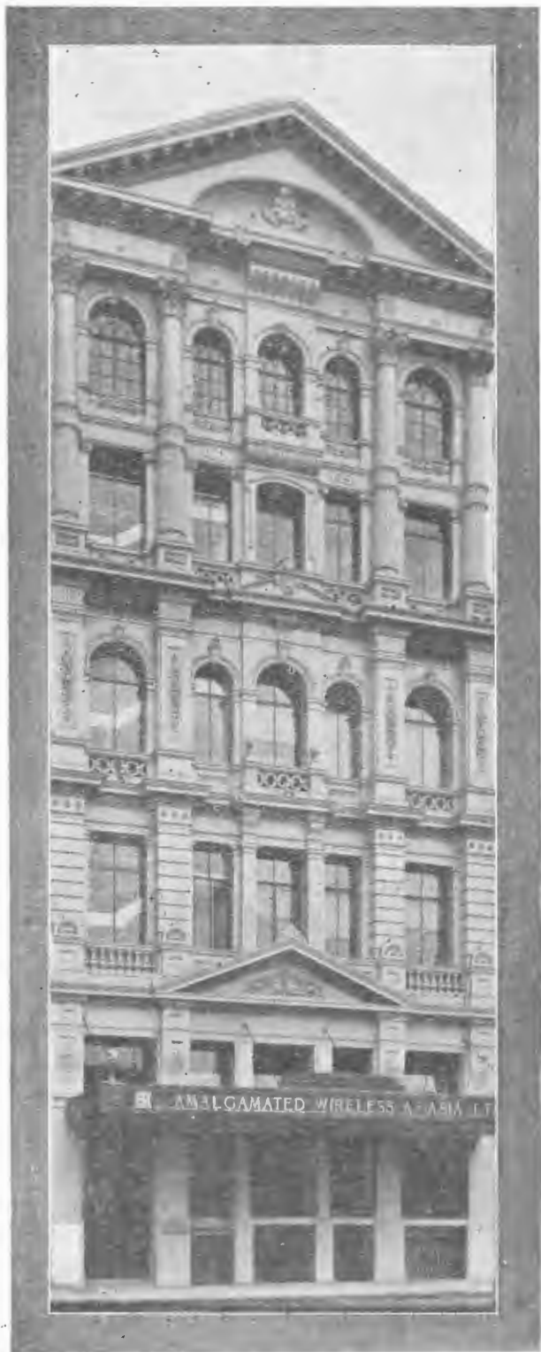
"Wireless House," 167-9 Queen Street, Melbourne.
