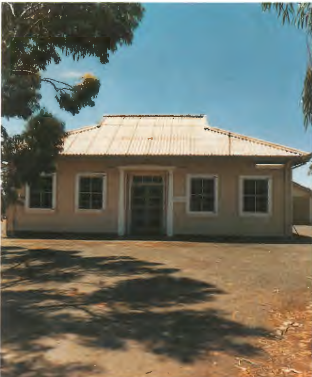
Original transmitter building erected 1936.
