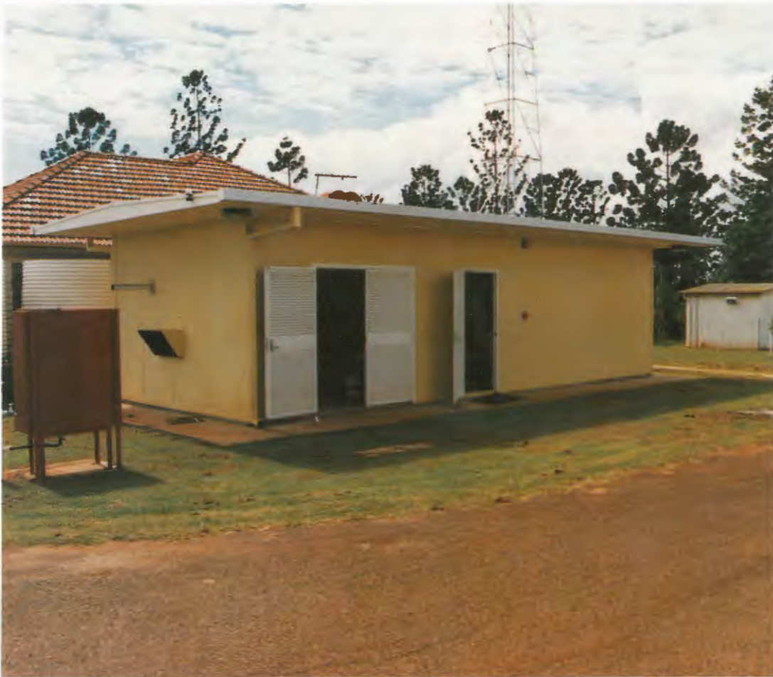
New transmitter building. Original building at rear.
