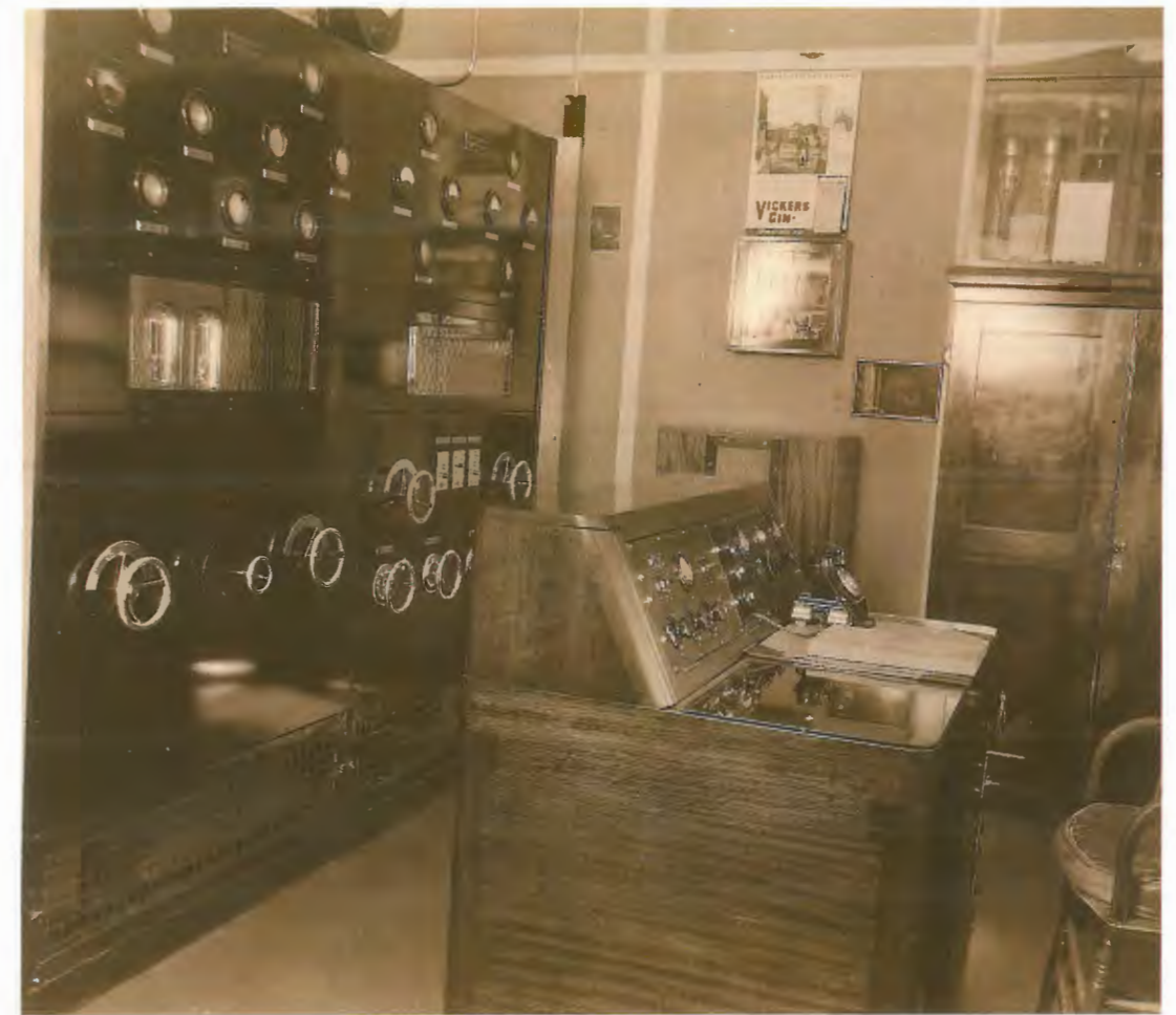
Original 2 kW water cooled transmitter installed 1931
