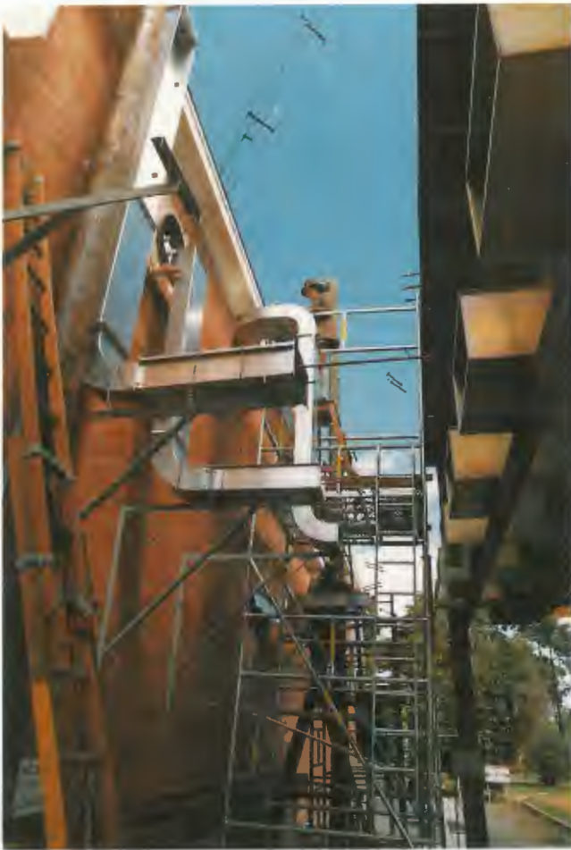
Doug Brodie and Lawrence Hester installing transmitter trunking.
