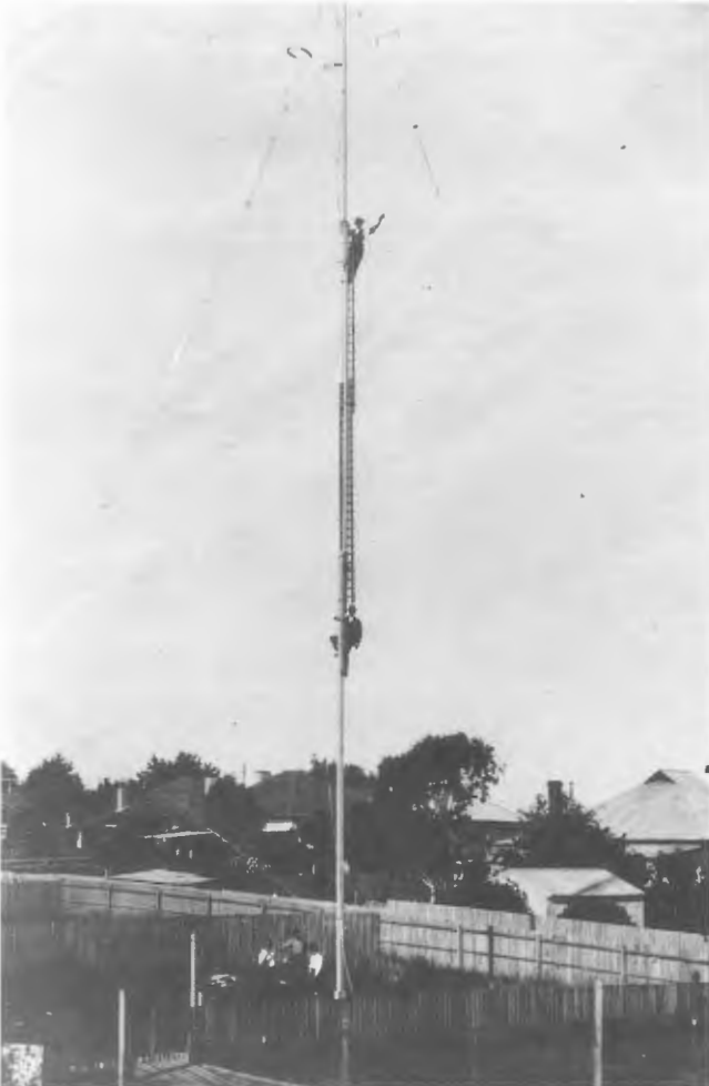
Stan Hosken (at bottom of ladder) with friends inspecting his 102ft (31 m) aerial used with station 3MP which began operation in 1924 on 219 metres (1370 kHz).
