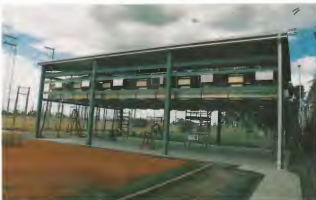
View of switch showing six antenna outlets.
