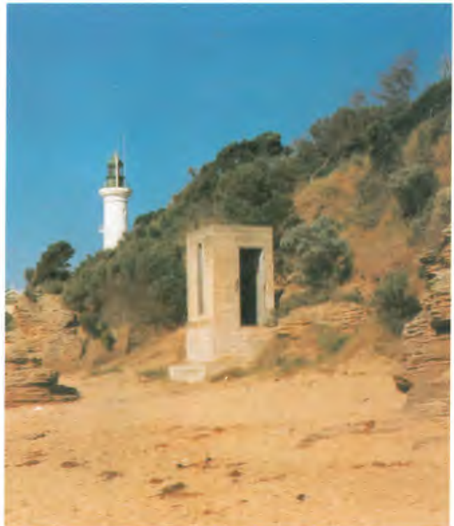
Infra-red bunker Point Lonsdale and lighthouse.
