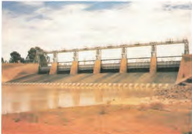
Weir on Darling River at Pamamaroo.
