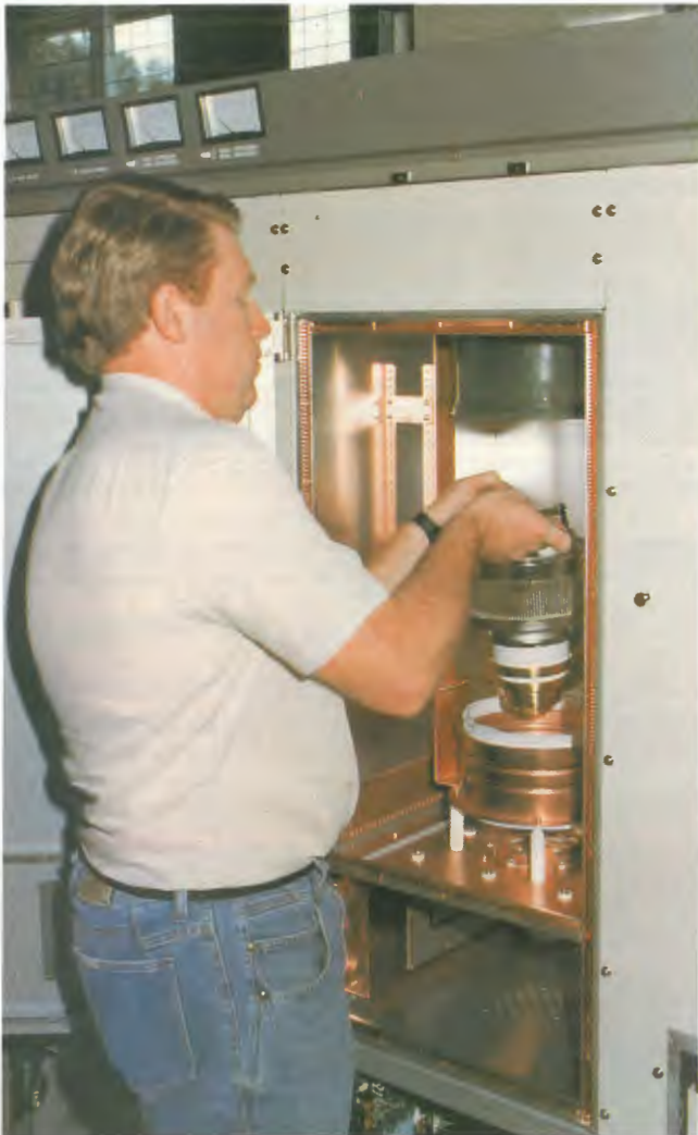
Alf Blackley inserting tube into cavity of new Channel 2 transmitter.
