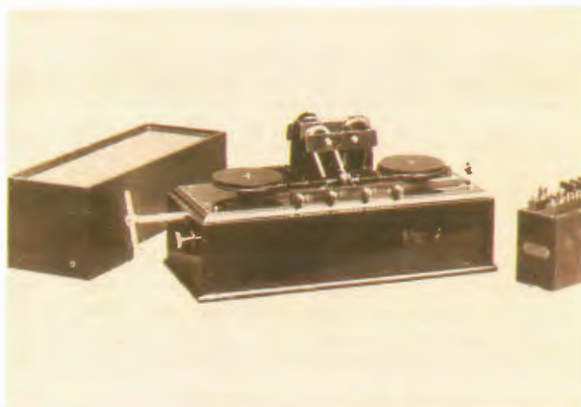
Marconi's magnetic detector which employed the effect of HF oscillatory currents on the magnetic properties of soft iron (Courtesy The Marconi Co. Ltd).
