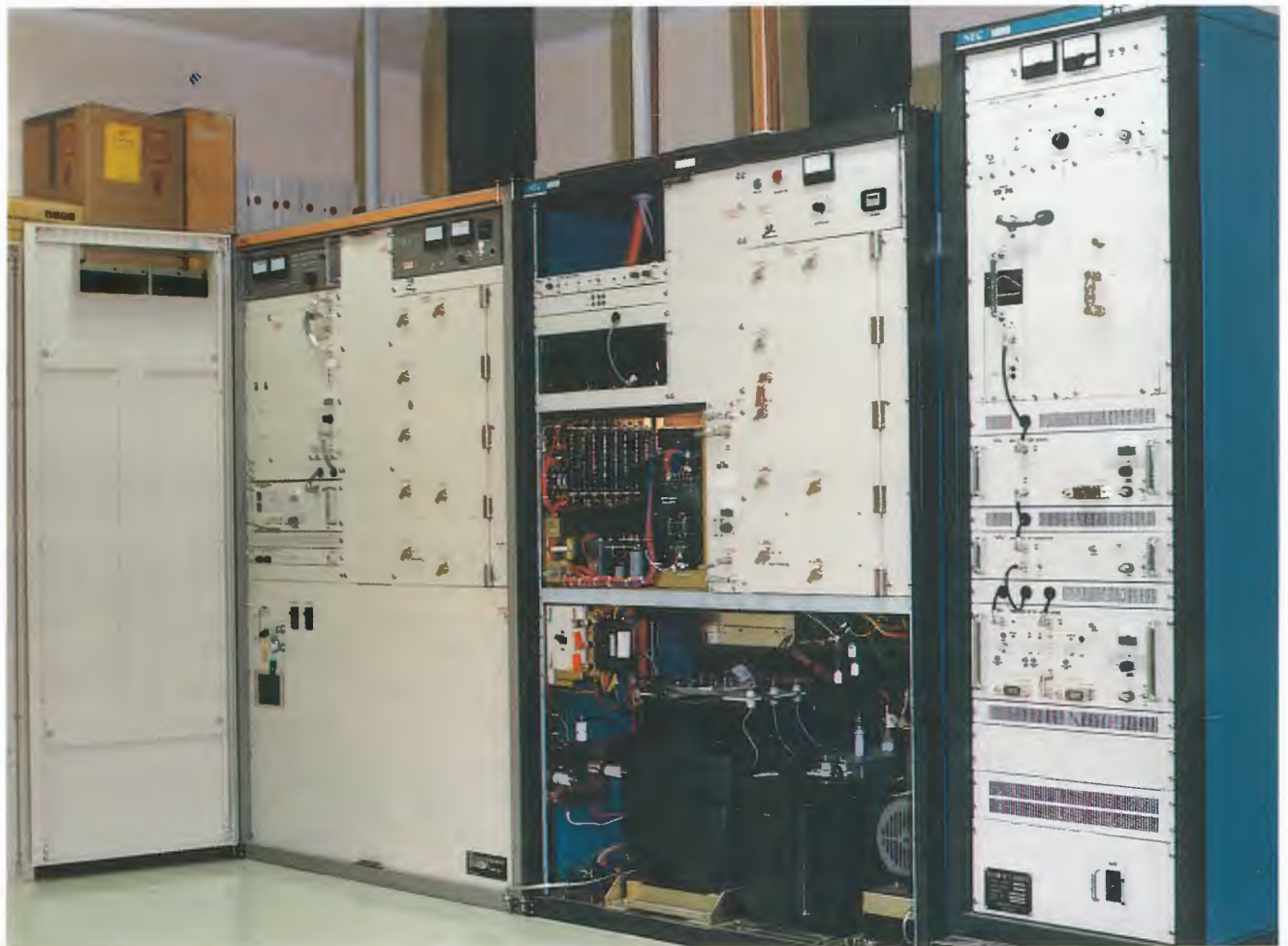
Some of the FM and TV transmitters at the Centre.
