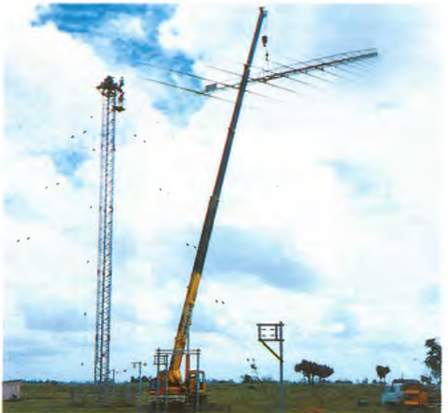
Log periodic antenna being re-erected following repair.
