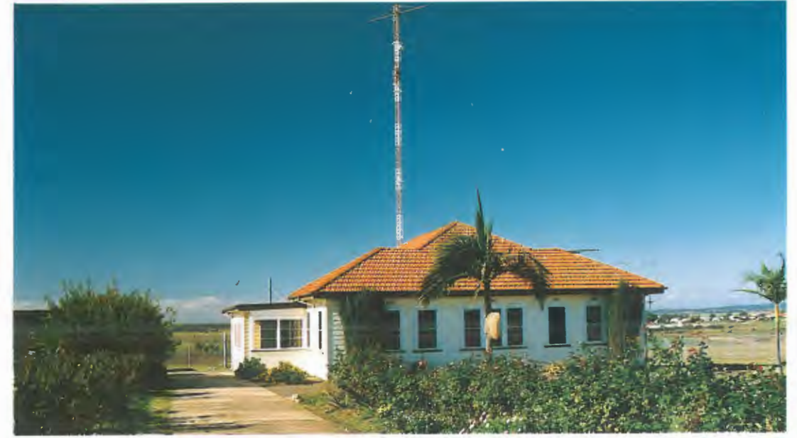
2NC building and main radiator.
