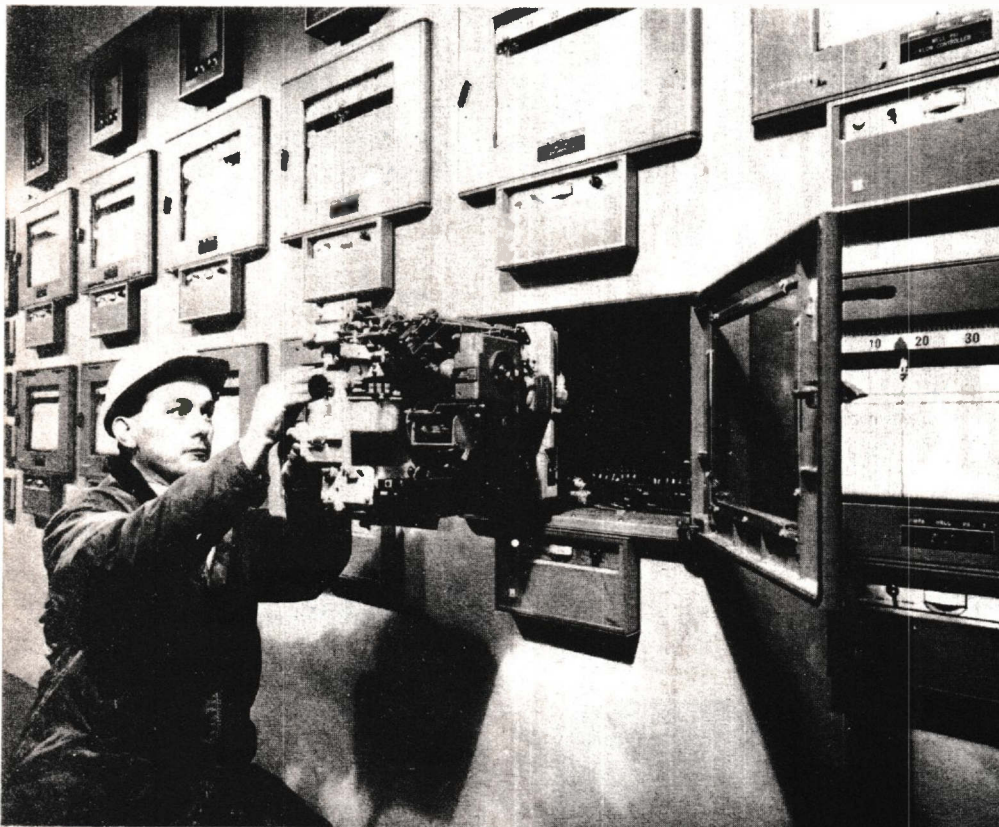
Fig. 1. Chart recorders are used in many varied applications. The panels of this control room contain a number that are used by the operators to see how the process is behaving.
