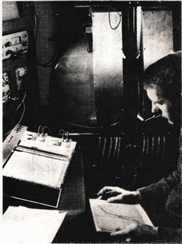
Fig. 4. Plotting a hysteresis curve for material under test in the large magnet shown at the rear.
