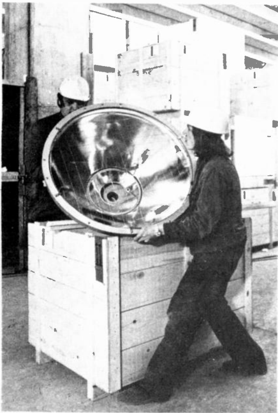
Seen here is one of the 550 metal halide vapour lamps used in the main stadium. Each lamp draws 28 kW.
