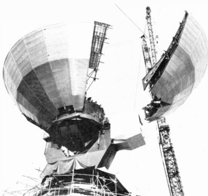
Third antenna currently being fitted to the Raisting Satellite Earth Station will send colour TV pictures around the world.
