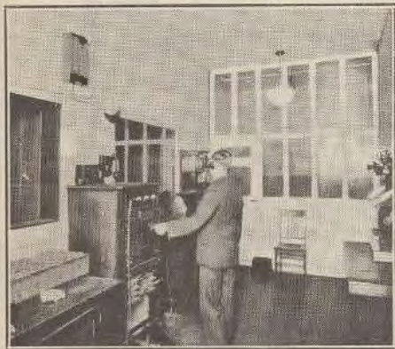
The Control Room at 2FC.
