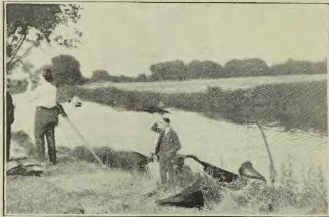
Erecting a Riverside Aerial
