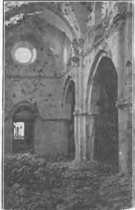
AN OBSERVATION POST OF THE ENEMY'S, WHICH MADE AN EXCELLENT TARGET DURING A BOMBARDMENT. THIS VIEW OF THE INTERIOR WILL TESTIFY TO THE ACCURACY OF THE GUNNERS.
