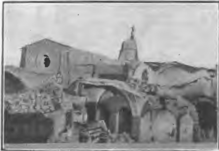
ANOTHER BUILDING WHICH WAS A GOOD TARGET FOR THE ADVANCING FORCES.
