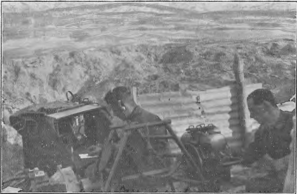
WIRELESS MEN AT WORK IN THE TRENCHES.
