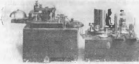
EARLY TYPE OF MARCONI TRANSMITTER.
