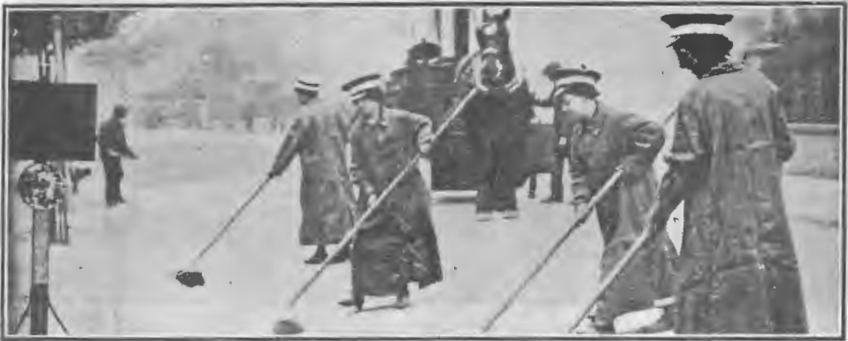
AT WORK ON THE ROADS IN A LONDON SUBURB.
