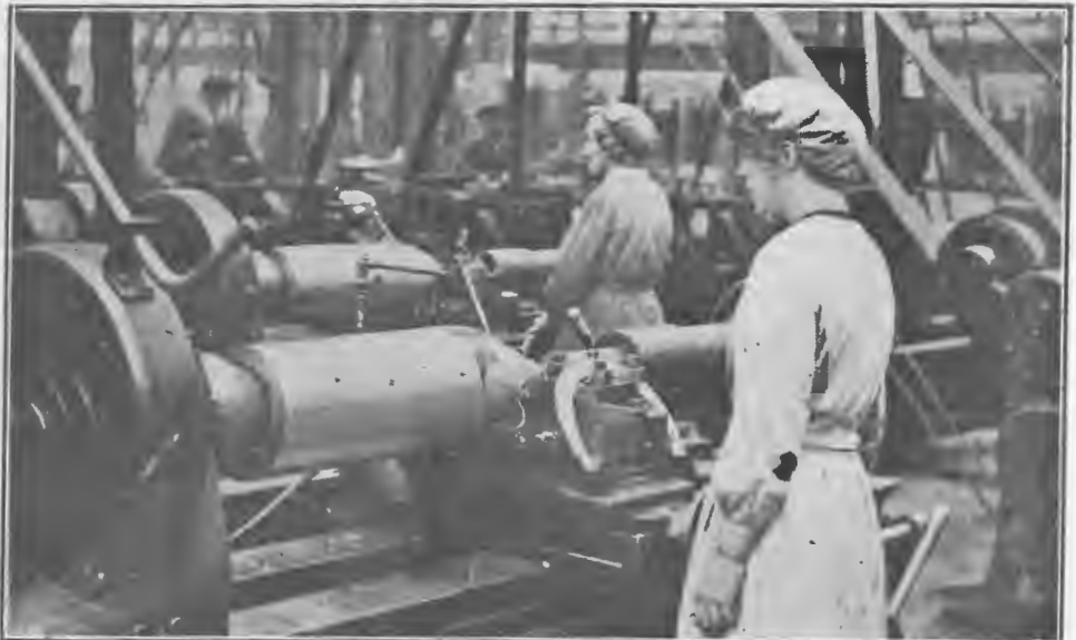
ROUGH-TURNING A SHELL IN A MUNITION FACTORY.
