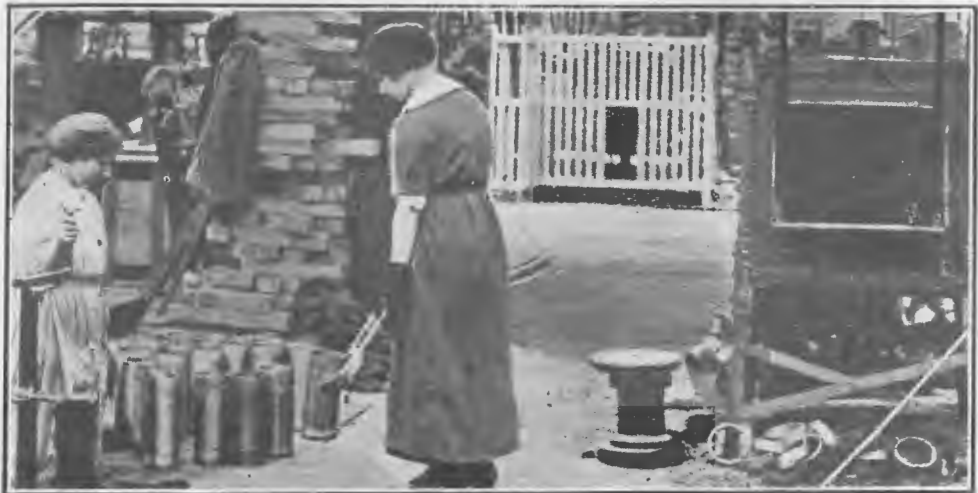
COPPER-BANDING 60 POUND SHRAPNEL SHELL.
