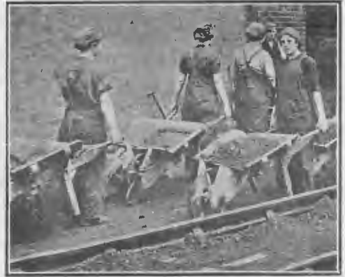
CLEARING EARTH EXCAVATED FOR THE INSTALLATION OF HYDRAULIC PUMPS.
