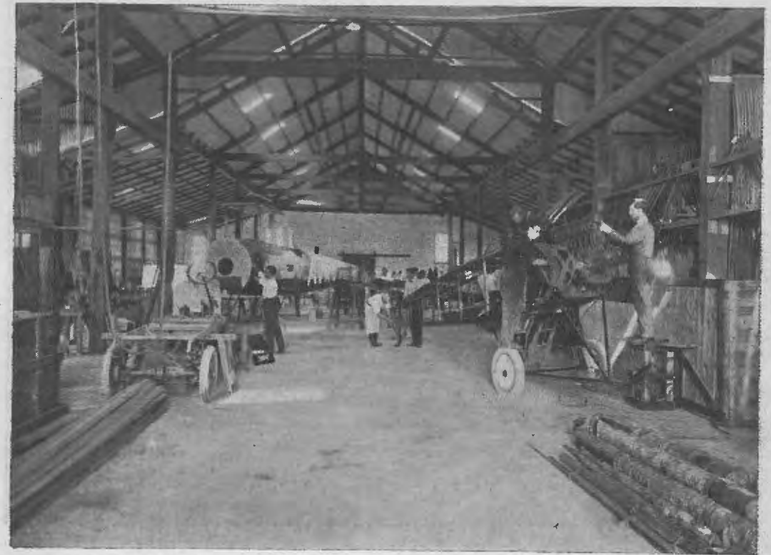
General View of the Assembling Shop at the Mascot Works.
