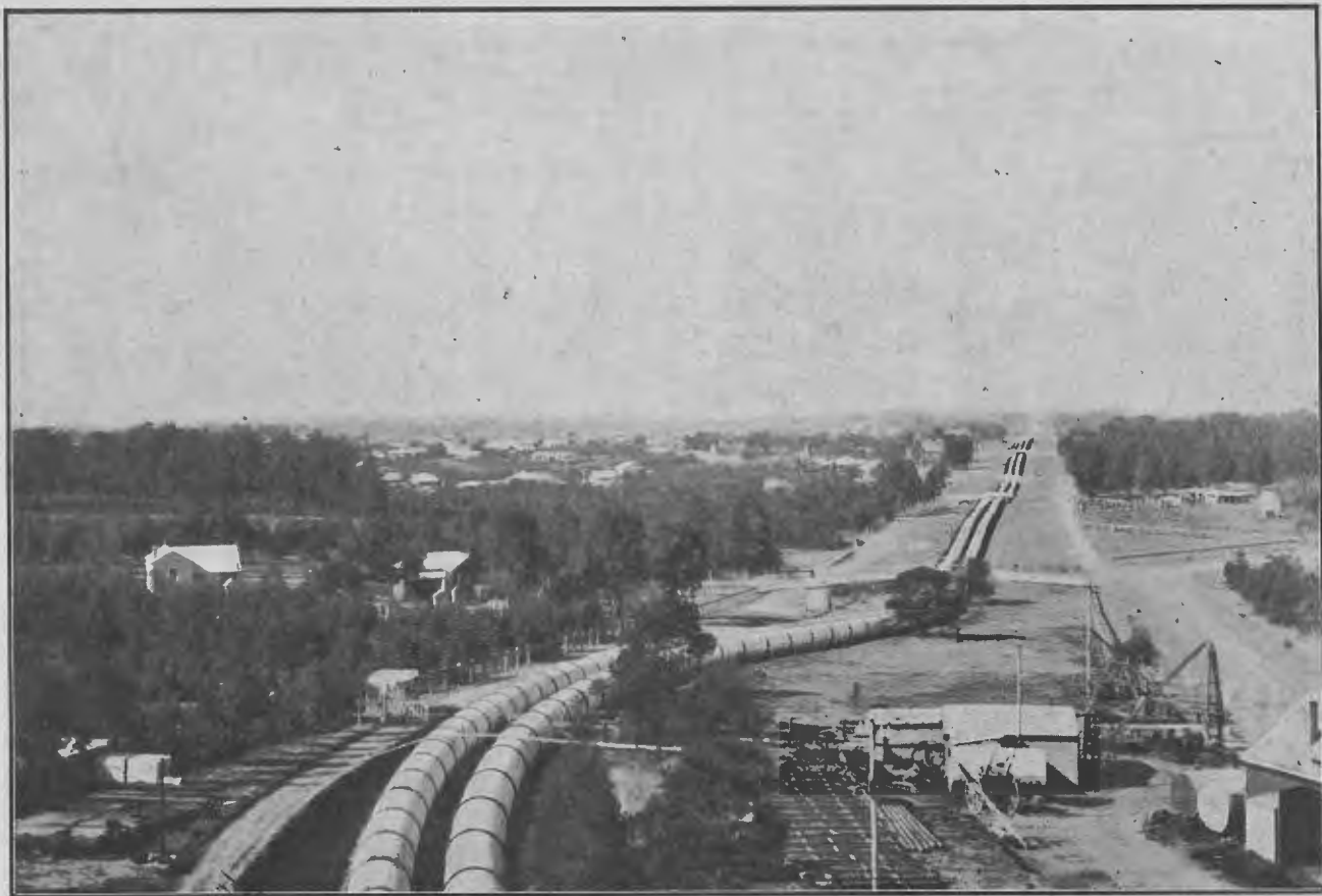
Pipe Line—Pipe Head to Potts' Hill.
