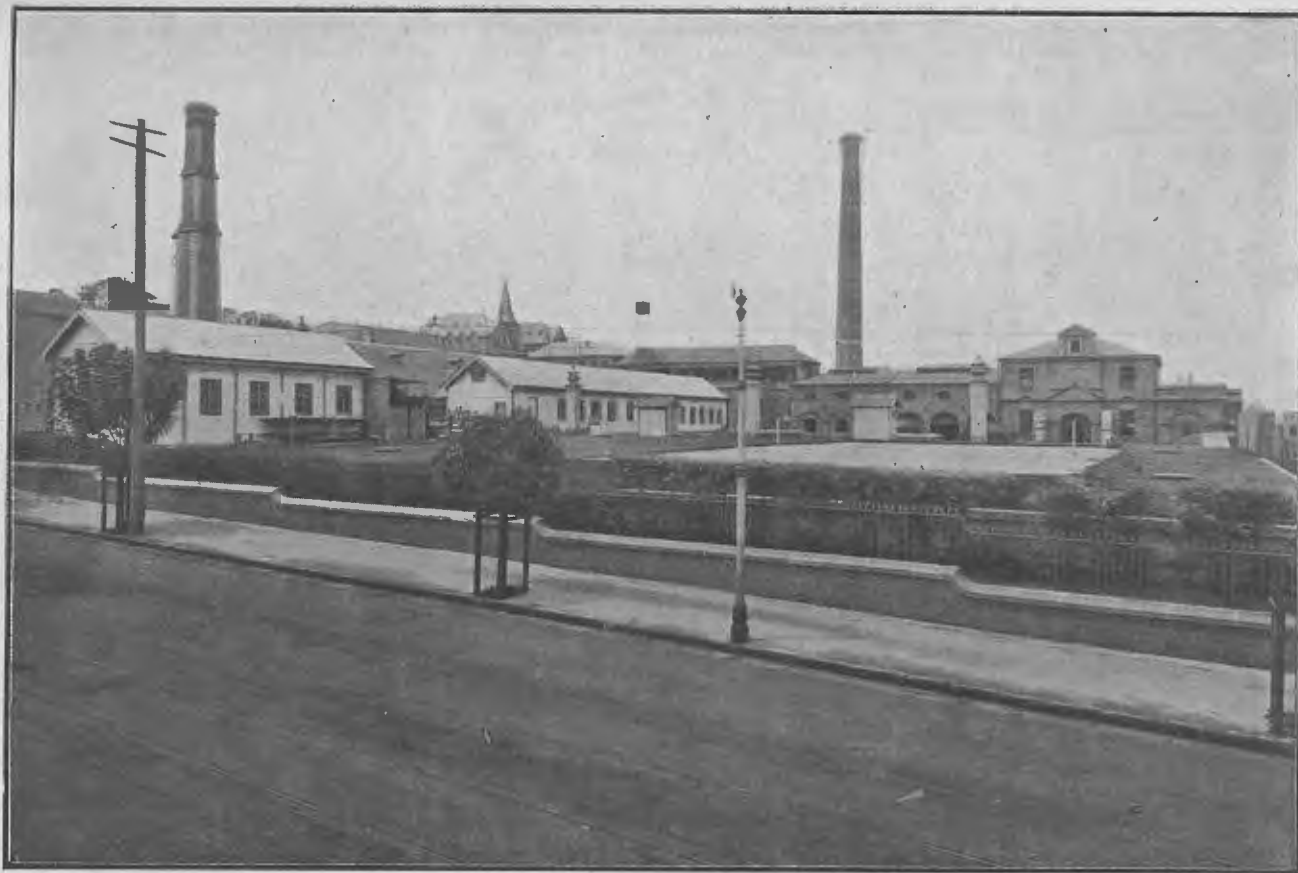
Crown Street Pumping Station and Works.
