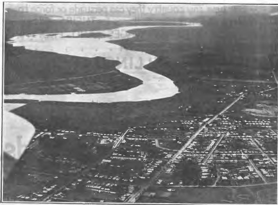
Aerial View of Invermay (suburb of Launceston, Tasmania) and River Tamar, photographed from Lieut. A. L. Long's Boulton and Paul biplane.
