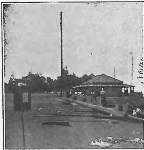
Ready to Erect the First Mast.
