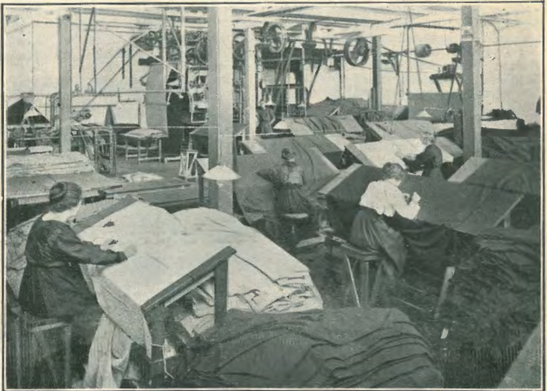
The Finishing Touches.
