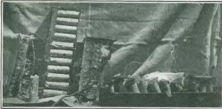
Re-built H.T. Batteries.
