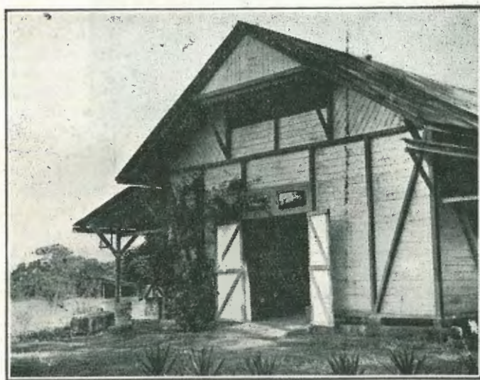
This is Kaewieng Radio Station, New Guinea. A 1½ Kw. Marconi transmitter is installed and a considerable amount of traffic is handled by this far outpost of the Empire.
