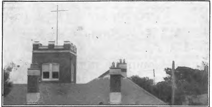
Aerial at 2DS. The tower on which the aerial mast is erected houses the radio equipment. (See diagrams page 428.)
