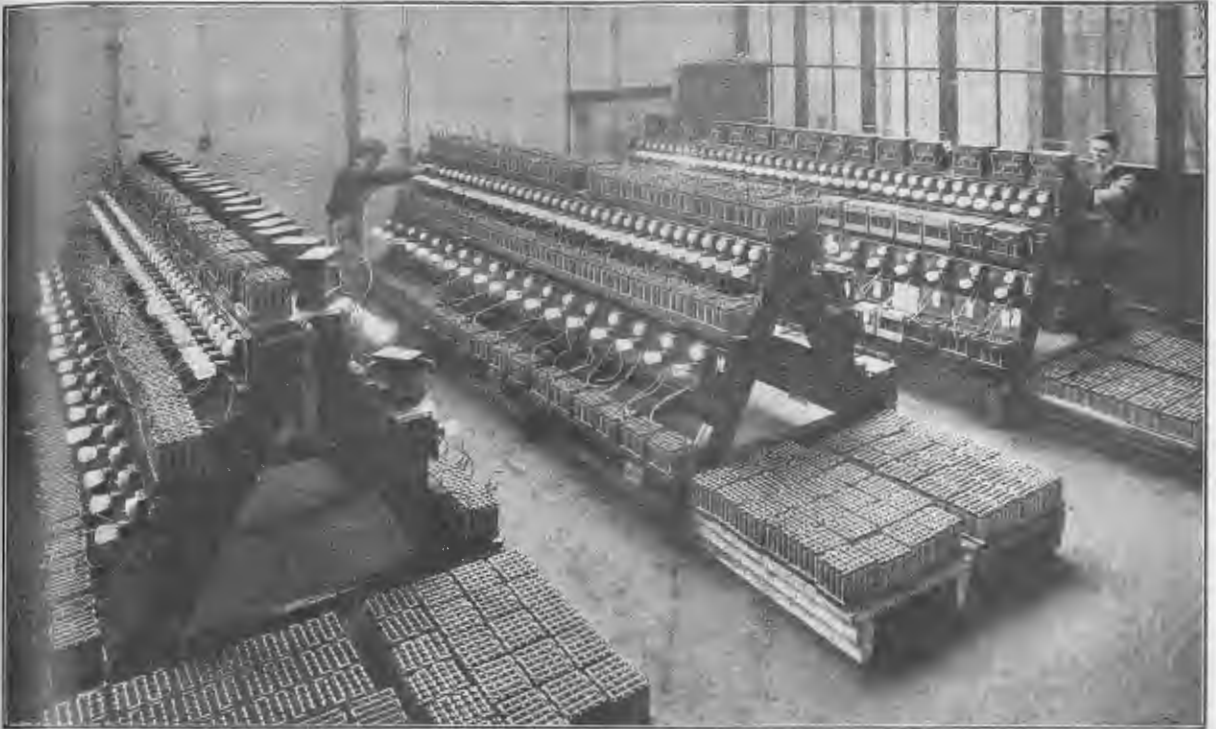
The H.T. Charging Shop at the C.A.V. Battery Works.
