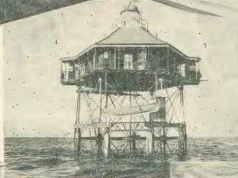
The Pile Light, Moreton Bay. It was near this spot where the descents were made.
