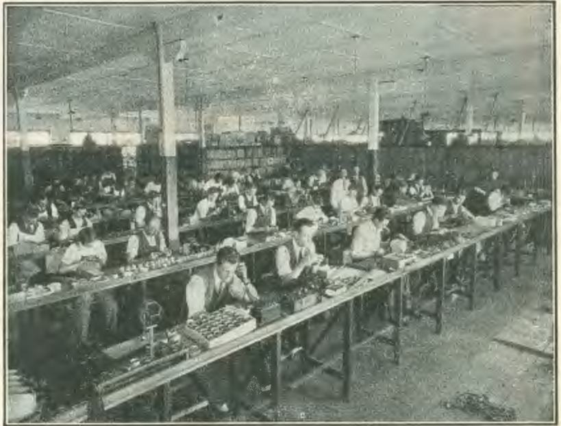
Section of Assembly Department.
