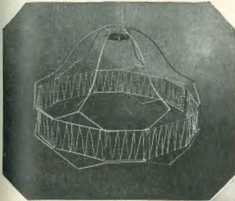
The uncovered lamp-shade frame, showing aerial frame inserted and bakelite lamp-socket holder.
