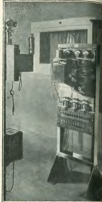
THE CONTROL PANEL.
