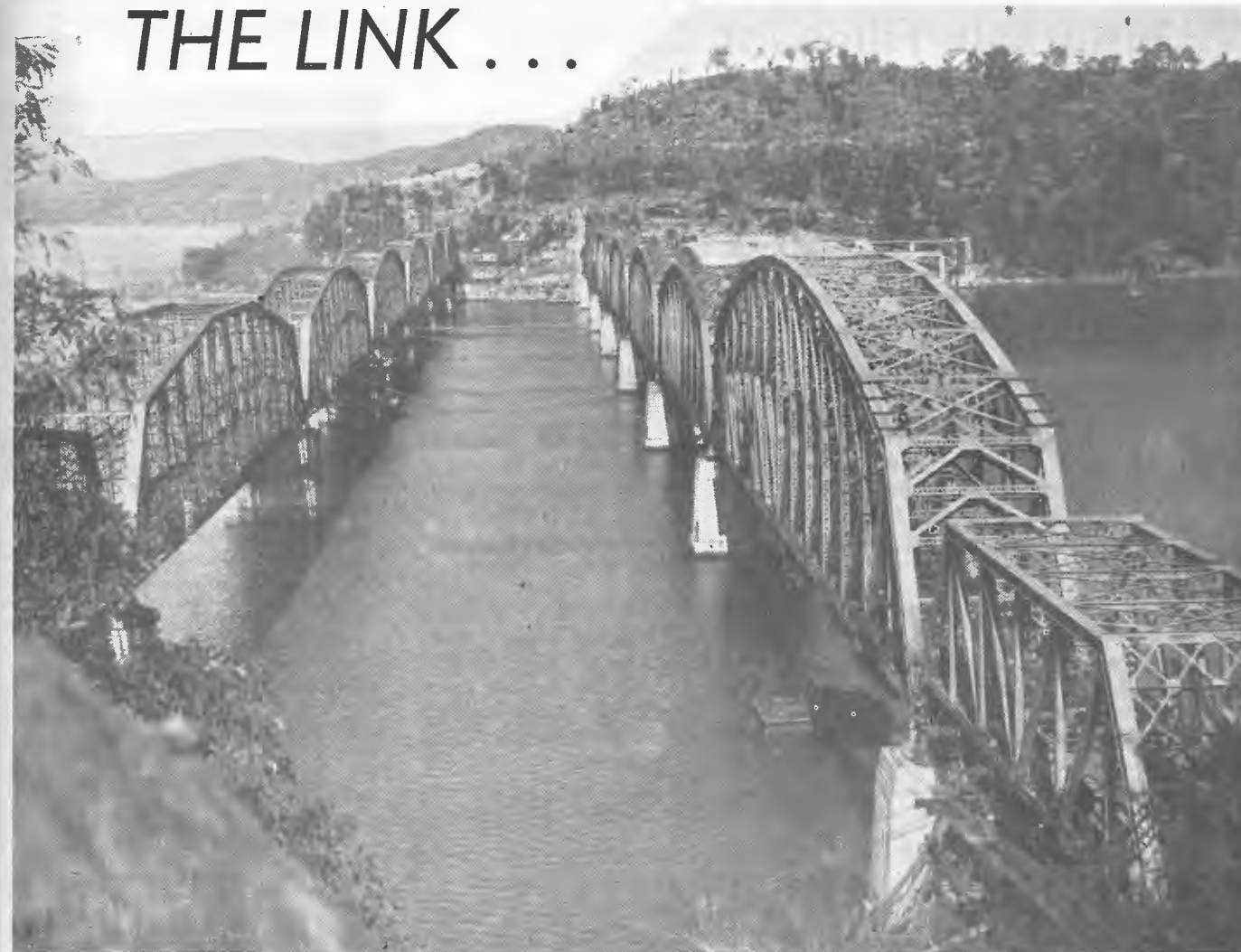
OLD AND NEW HAWKESBURY RIVER BRIDGES
