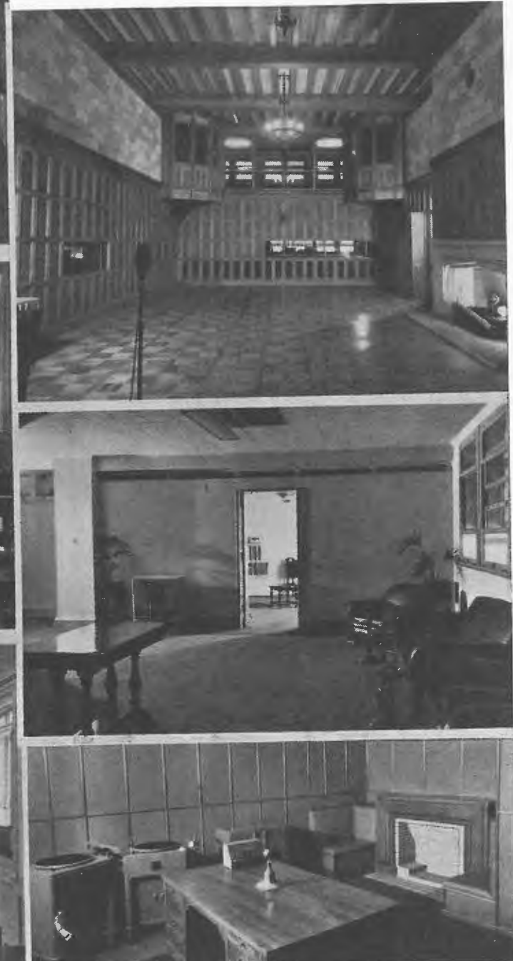
The new 2CH studios on the 11th floor of the A.W.A. Building, Sydney, are now being used. They represent the most modern development in construction and equipment as indicated by the above pictures. Top left shows a view of the main studio with seating accommodation and showing the special flooring fitted in sections. Each section rests on pneumatic tubing which assists in the acoustic regulation at any point according to pressure applied. Centre left: View of same studio looking down from the foyer on the 12th floor through three layers of plate glass and showing seating accommodation, placing of microphones and general arrangement for audience participation broadcasts. Note the large fireplace at left. Bottom left is a view of No. 2 studio on 11th floor. This studio is normally used for all 2CH programs. Equipment includes a special four-position transcription turntable fitted with the latest type R.C.A. pickups and a closeup of which is shown elsewhere in this issue. Top right: Main Studio again, looking east towards the foyer (top background). At centre left of this picture can be seen the producers panel window. Centre right: In the foyer on the 12th floor with No. 1 Audition room in the distance. Foyer is used by sponsors to view and hear big programs broadcast from No. 1 Main Studio, on 11th floor. Bottom right: No. 3 studio on 11th floor, used mostly for talks and programs controlled by special announcers. Equipment includes two of the latest type transcription units for program or audition discs.
