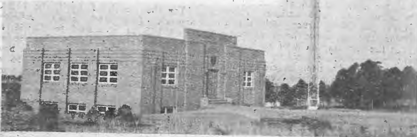
2SM's new Broadcast Transmitting Hall and half-wave radiator—the only one of its kind in operation in Australia—located at Pennant Hills
