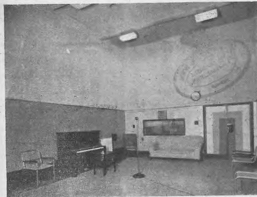
Portion of 3AW's Studio A, in Melbourne. This studio is on the street end of the building and is large enough to accommodate a band of 50 players. The Studio measures 28 feet x 17 feet.
