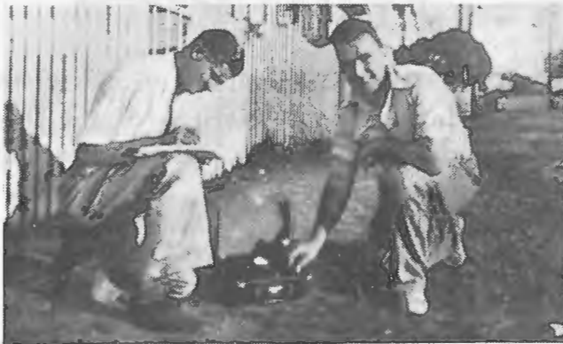
Left: VK4RF (left) and his co-experimenter, VK4EL, making field strength tests while trying out a special type of matched impedance vertical antenna.
