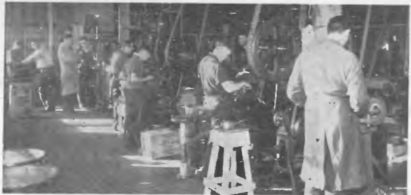
Below are shown the large power presses which form part of the machine shop equipment. They are used to stamp out all pressed metal parts used in Crown products.
