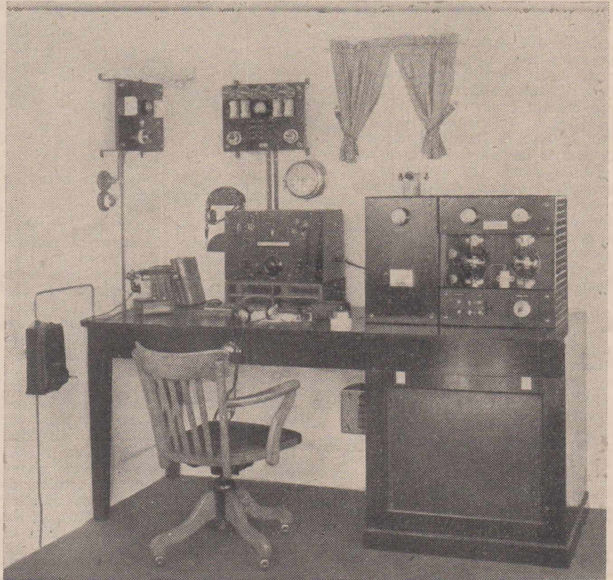
● This was a marine radio installation of the 1920's. The sea-going operator of the 1950 era has much more comprehensive equipment under his control, especially on the larger vessels.
