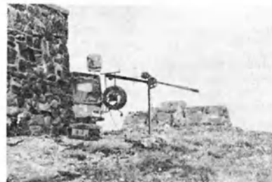
Wind Generator. Mount Hotham.
