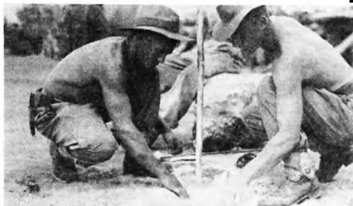
Boring holes in Morotai Island. They did actually do this through the coral crust to "great nothingness."
