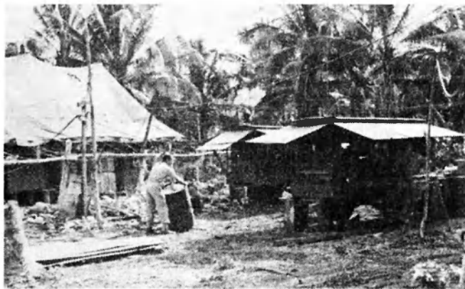
Original 'Landops' transmitter shack at Morotai — a leaky marquee with two 25 kVA alternators (Ford Mercury) outside.
