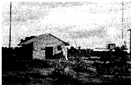
The temporary W/T station, situated at Parap.
