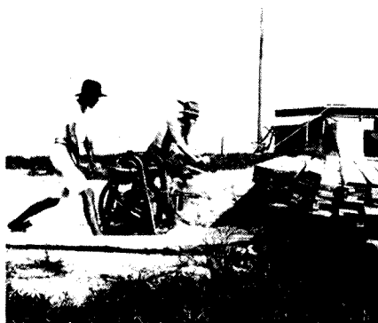
Winching up timber from the beach
