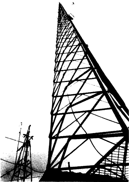
Dural's antenna towers. Left is the 12m tower with beacon and 6m antennas; right is the 30m tower with 70 cm and 2m repeater antennas and link antennas.
