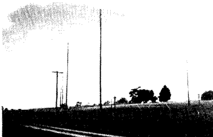
Antennas from the roadway
