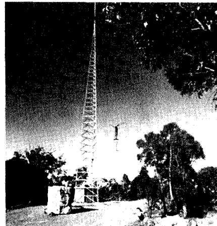
Photo shows the repeater site.
