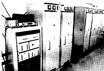
Three J54800 AM transmitters with matching power supplies. Far left is a rack containing beacons with 6 and 2m SSB transceiver on top.
