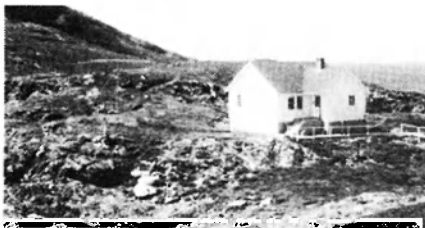
The shack and beam (Note: the rocky terrain)
