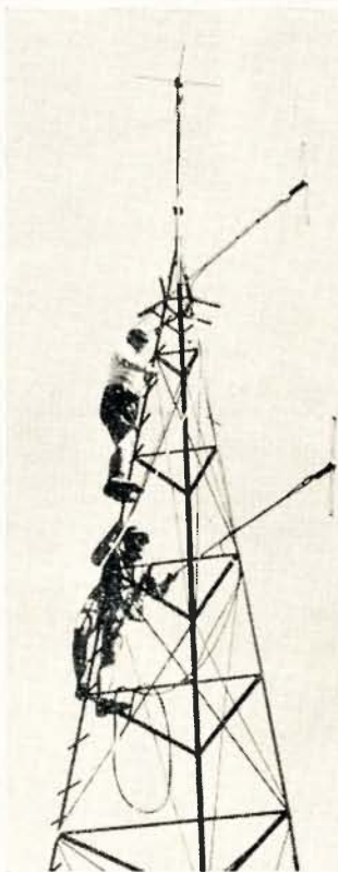
Aerial phasing.—The ground plane is part of a commercial system located at the same site.
