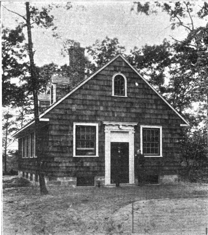
RIVERHEAD RECEIVING STATION
