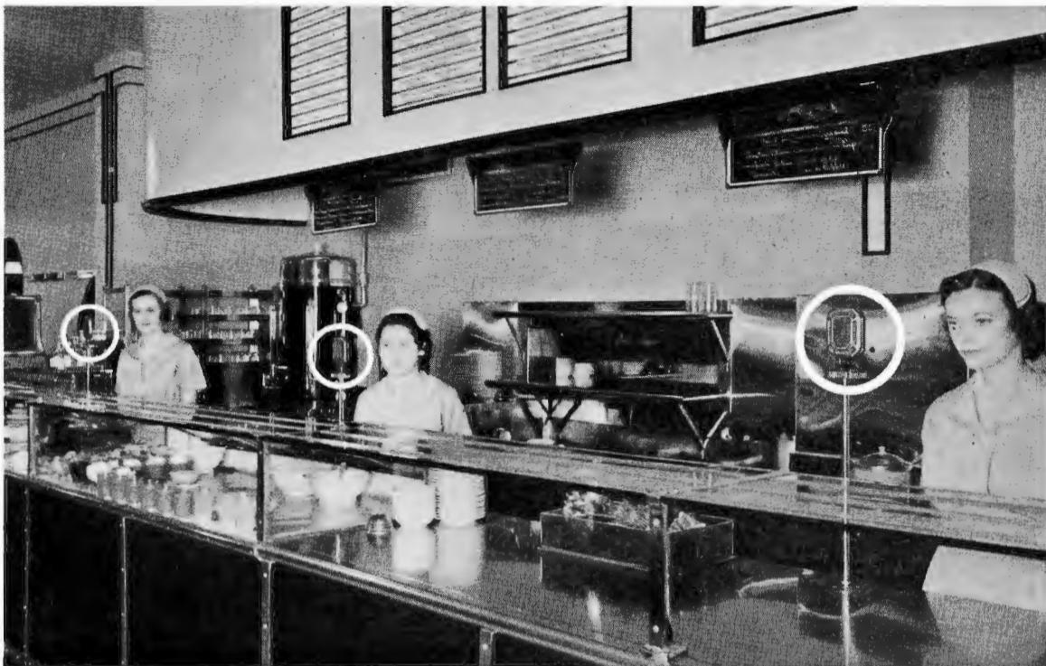
The Franklin Cafeteria of Hartford, Conn., speeds its service to customers through the use of an RCA PG-63 Public Address System operated with three carbon microphones. Microphones placed on the counter permit attendants to pass orders to the kitchen through the use of a loudspeaker and amplifier.
