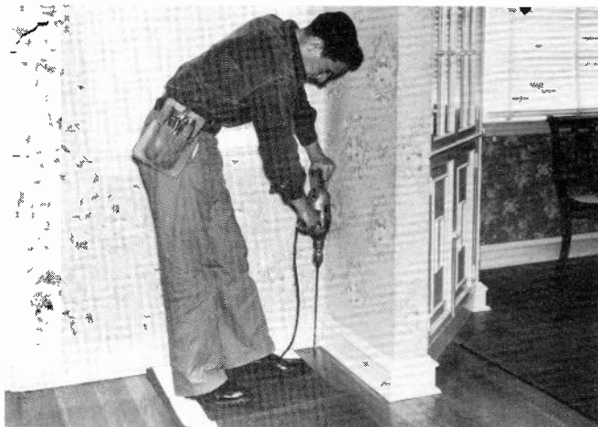
If an electric drill is used, make certain that it is grounded.
