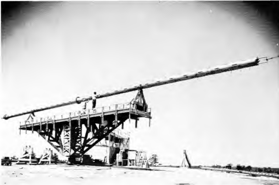
TESTED at RCA's facility at Gibbsboro, N. J., this powerful TV broadcasting antenna was shipped to WSBT-TV, South Bend, Ind.
