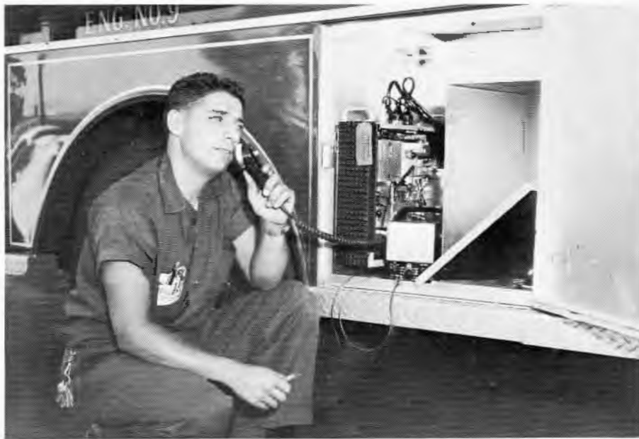
TPS Tech Pete Cerruto checks a Newark, N. J., fire engine unit.
