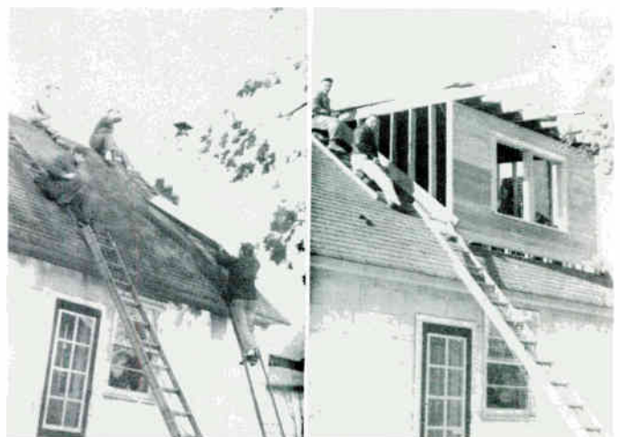
Three Flushing techs, J. Hodgson, T. Humble and A. Kauth, put their collective ladder experience to good use when they helped J. Kobbe put a 12-ft. dormer on his expansion attic—completing the large order in only one day!
