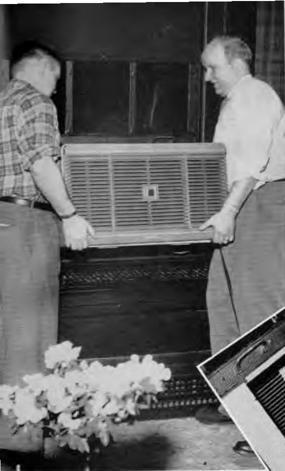
MANHATTAN journeyman tech Walter Scheck (r., above) and tech Bill Brey insert cooler in window of Park Ave. apt. (Right): Scheck secures brackets
