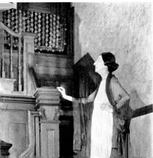
THIS IS LIVING ROOM STAIRWAY
