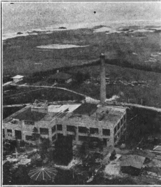
POWER HOUSE—OCEAN, IN BACKGROUND
