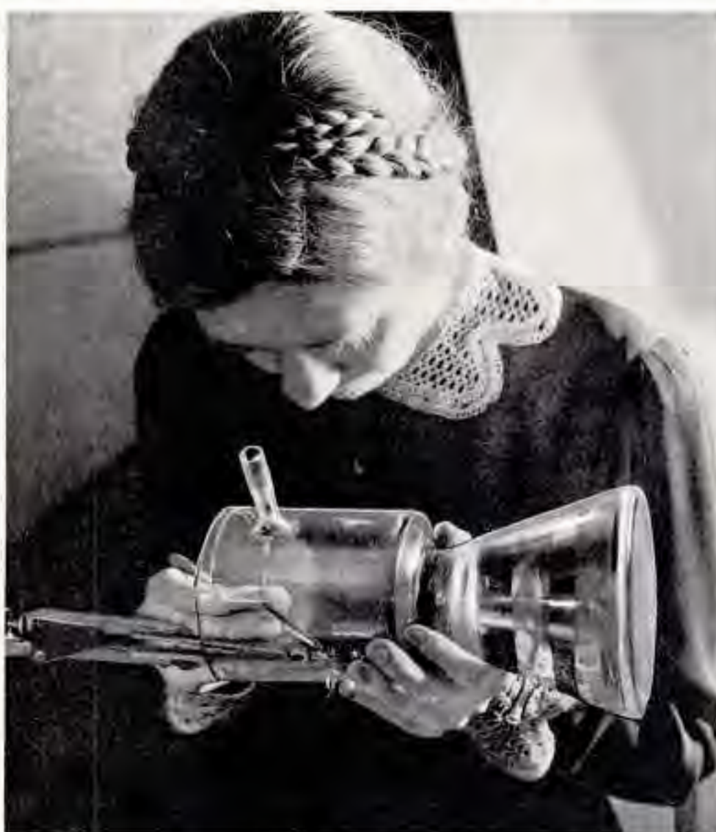
Nimble fingers are needed in putting together the intricate "innards" of many types of RCA vacuum tubes used in radio. Above is Christine Swenson, one of the many skilled workers at the RCA radio tube plants in Harrison, N. J., and Indianapolis, Ind.
