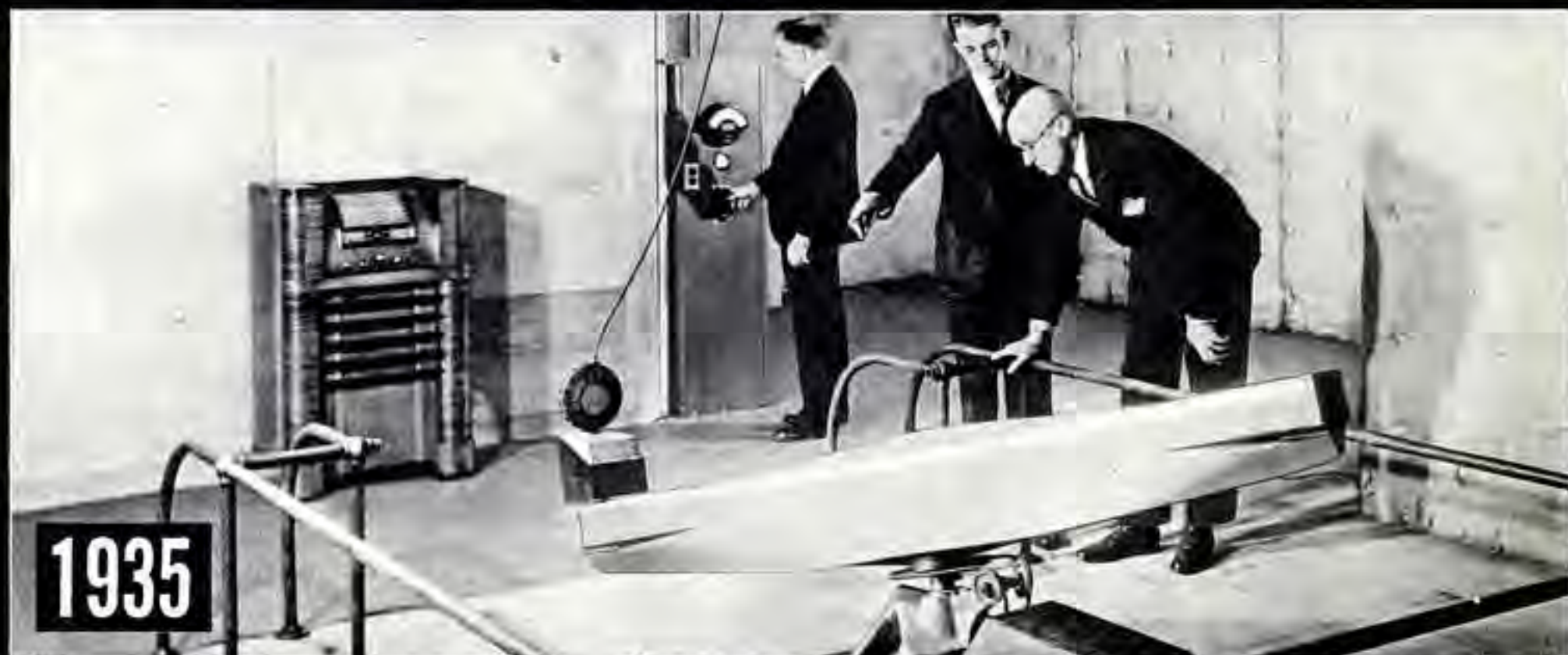
THE BIRTH OF THE MAGIC VOICE —Seeking for tone perfection RCA engineers seal speaker chamber and install group of tone pipes which trap "boom" and end distortion. Named MAGIC VOICE , this advance justifies its title under test by "Electric Tone Detective" shown above with 1938 model. More accurate than human ear this RCA-designed tester automatically records tone performance.
