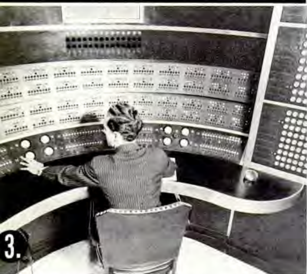
The cross-roads of the air —The artist's voice and Mr. Black's music are now ready for the NBC Blue Network. The entrance to this (and also to the Red Network) is through the giant switchboard shown above. The operators at this board turn their particular RCA Magic Keys and the Magic Key goes out to the NBC stations which carry it. A complete duplicate of this switchboard provides for emergencies.
