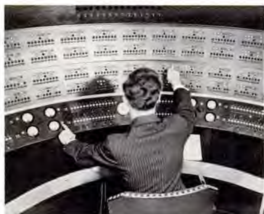
RADIO CITY —From Riverhead, program is relayed by wire to RCA Communications, 66 Broad St., N.Y.C. It is amplified there, and despatched over another wire to the NBC Master Control Board at RCA's Radio City, explained in detail on two preceding pages.
