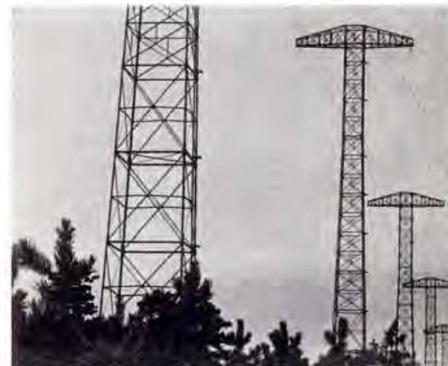
RIVERHEAD —Program is received on these great antenna towers at RCA's Station at Riverhead, L.I. This important link in chain covers 1½ square miles. From its transmitting station, at nearby Rocky Point, RCA sends Radiograms, 200 words per minute, all over world.
