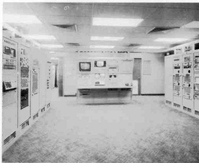
Fig. 5. Aerostat ground station. Cabinets on the right contain the MTI processor and radar telemetry and the synchronizer/demultiplexer subsystems. The radar and telemetry operating consoles are in the center. They are configured to support two-aerostat operation. Racks on the left contain equipment for monitoring and controlling other aerostat systems such as pressurization and power generation.
