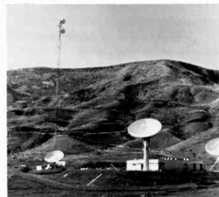
Fig. 5 Ground facilities such as these located at South Mountain, Cal., provide private leased-channel and tv services to major commercial centers. Each ground segment includes a CTO, a terrestrial microwave link, and a commercial earth station.
